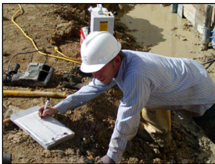
Fig. 12 Logging Pier Depth and Hydraulic Pressure
