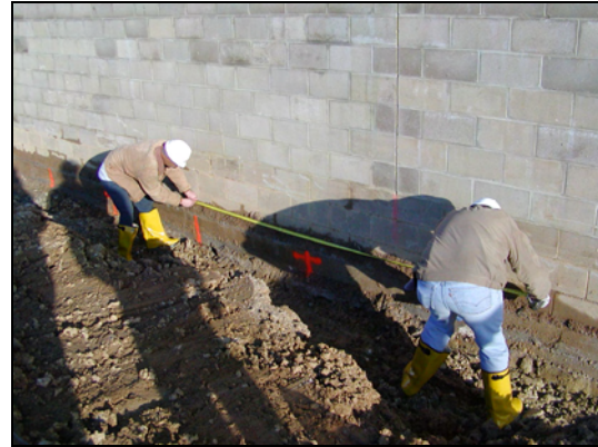
Fig. 9 Marking Bracket Positions Along Foundation Walls
