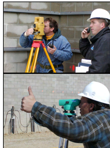
Fig. 13 Monitoring Wall Movement During Lifting Phase
