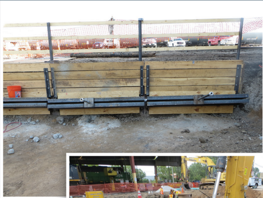
TYPICAL SECTION OF DRIVEN PIER & TIE-BACK ANCHOR 3/4" = 1'-0"
